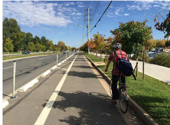
A separated bike lane in suburban Boulder, Colorado using posts & concrete curb stops as a physical barrier
