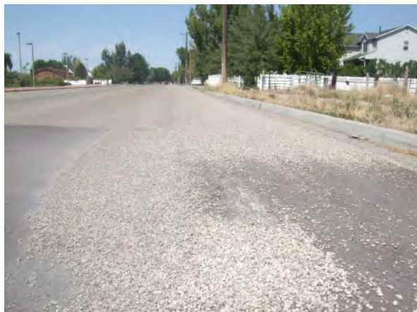
The chip size on an Angel Street project in Kaysville (pictured before resurfacing was complete) raised some concerns from residents and bicyclists (Photo: Shaunna Burbidge)
