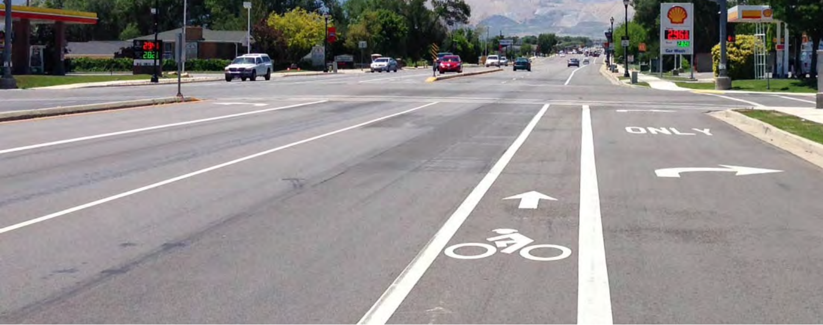
A through bike lane next to a right turn lane on a UDOT road in Salt Lake County
