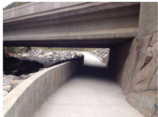
A grade-separated undercrossing in Logan, Utah that uses the existing slope and riverbed to pass under a roadway
