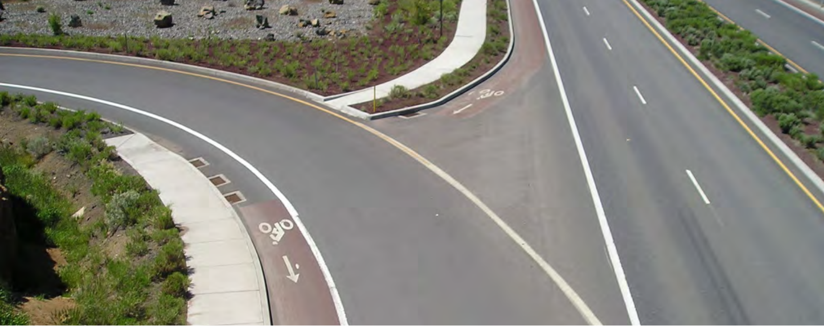
A bike lane crossing of a high speed, motor vehicle priority off-ramp near Hwy 97 in Oregon
