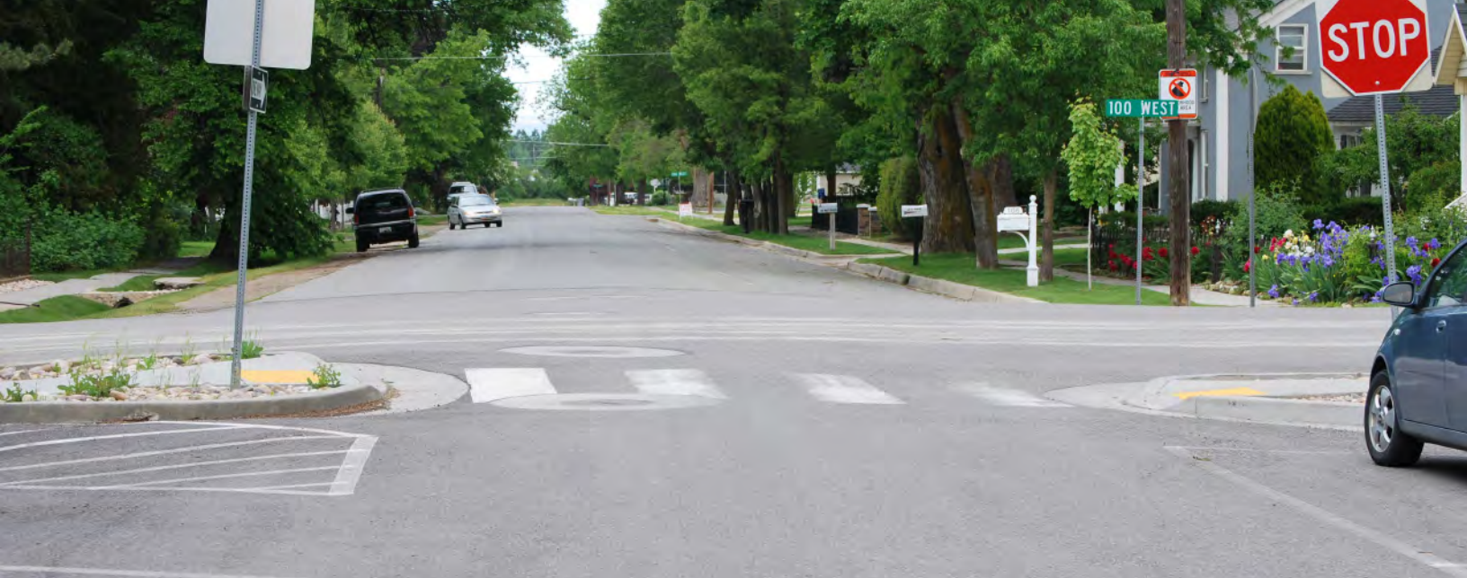
Curb extensions (or a choker or neckdown) at 100 West & Center St in Kaysville (Photo: Shaunna Burbidge)
