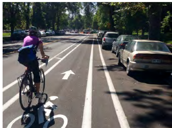
Buffered bike lanes have a painted buffer on the travel lane and/or parking lane side, based on volumes, speeds, and parking turnover
