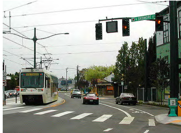
A "complete street" in Portland, Oregon, where bike lanes, travel lanes, parking, and light rail are all functioning in the same roadway right-of-way
