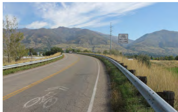
Shared lane marking and signage on Shepard Lane near I-15
