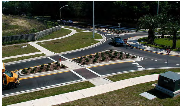
Roundabout improvements include curb ramps, marked, high visibility crosswalks, signage, and channelizers
