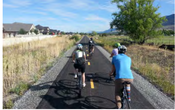
The Denver & Rio Grande (D&RG) Western Rail Trail shared-use path in northwestern Farmington near Burke Ln
