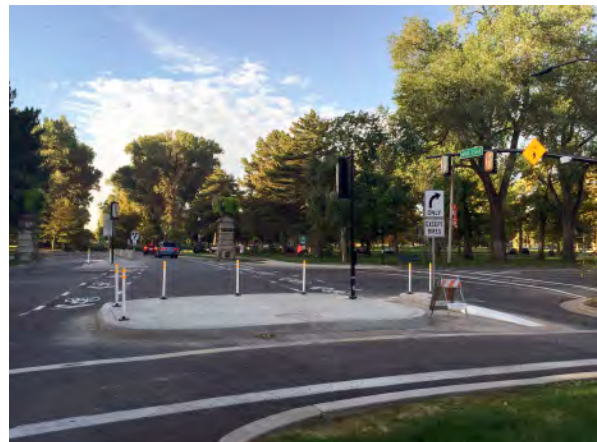
A TOUCAN beacon at the north entrance to Liberty Park in Salt Lake City. The TOUCAN was combined with a right-in, right-out treatment for motor vehicles, allowing bicyclists and pedestrians to enter and exit the park on 600 E while avoiding attraction of non-local traffic into surrounding neighborhoods.
