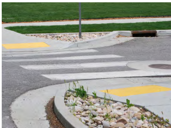
Curb extensions, shown here in a residential Kaysville neighborhood, shorten crossing distances for pedestrians and can calm traffic as well without reducing roadway capacity (Photo: Shaunna Burbidge)
