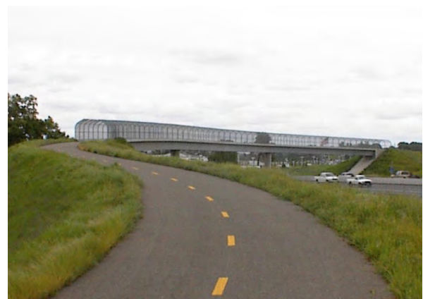
New bridges (overcrossings) should accommodate pedestrians and bicyclists, both on the structure and on the approaches
