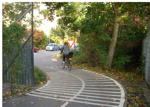
The above example shows a curve in the trail alignment that creates a near perpendicular crossing and perpendicular pavement markings that visually and tactilely slow trail users before the intersection. Creating an artificial curve in the trail alignment will slow trail users and improve crossing safety by bring the crossing closer to perpendicular to the roadway. Crossings should be, at a minimum, 60, and ideally, 90 degrees
