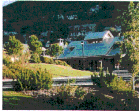
Sensitive grading and landscaping help this transit center building blend into its surroundings. (Park City, Utah)
