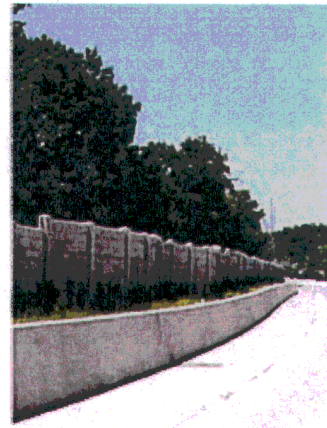
Solid sound walls that block views and access are not appropriate along Legacy Parkway.
