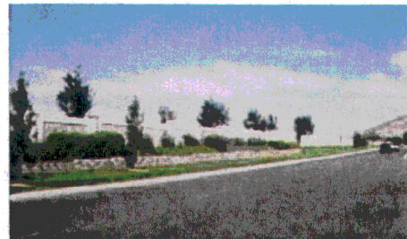
Tiered sound walls with berms, vegetation, and some wall sections that permit some views and access are recommended. (Farmington City's soundwall)
