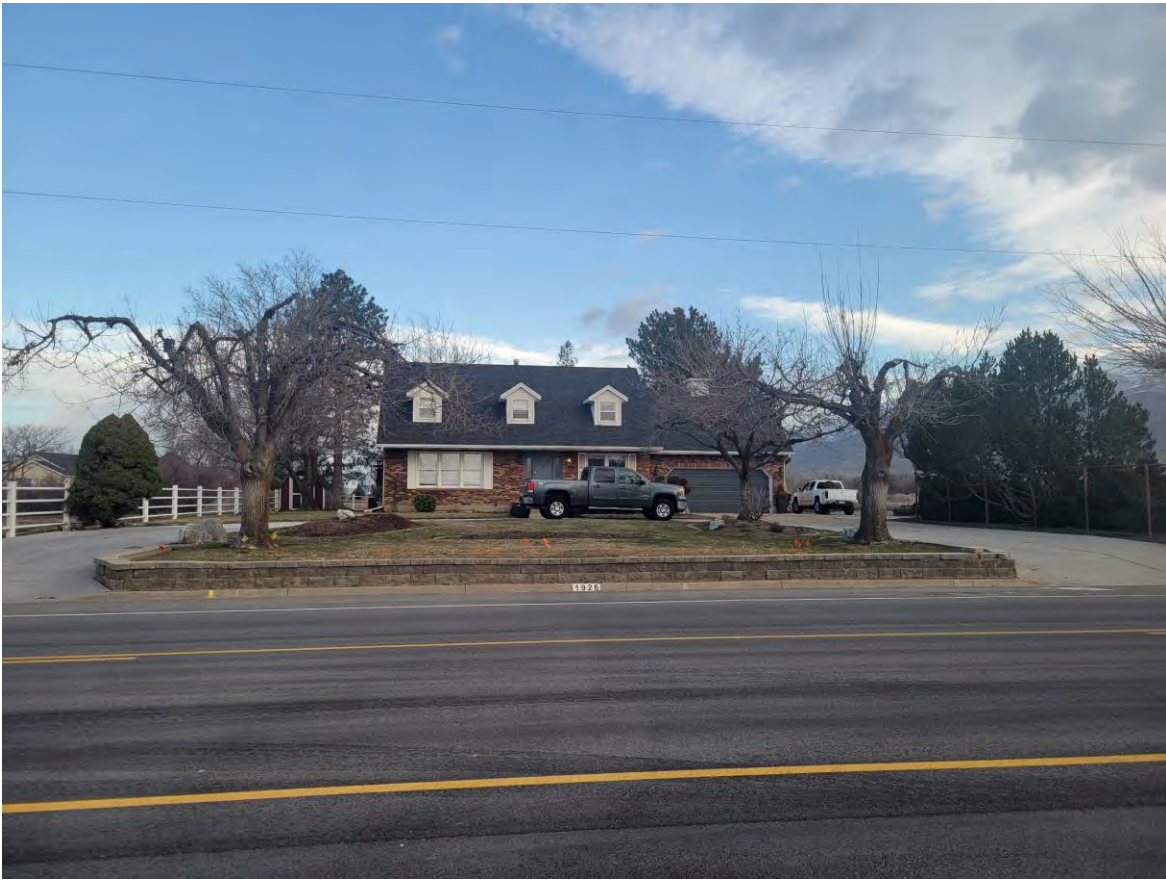
Existing Home – Retaining Wall, Ash Trees, Driveway Access
